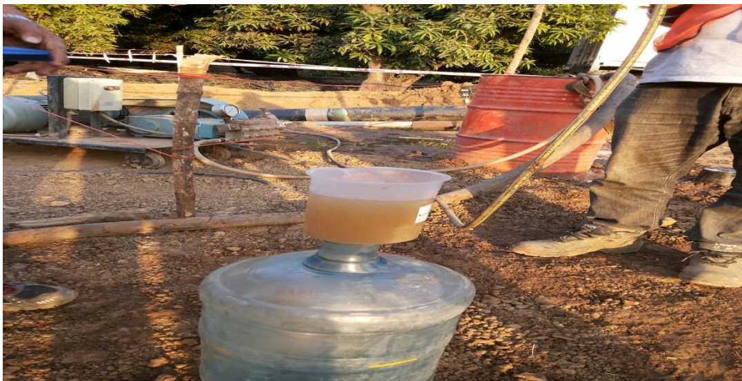
Figure Lowering of water
