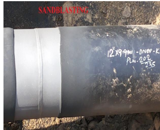
Figure Sand blasting
